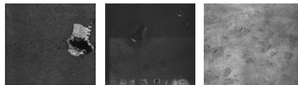
(a) Scale (b) Foreign material (c) Crack
